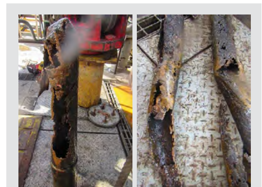
Figure 1: Recovered corroded tubing.
