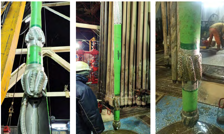
Left: Whipstock assembly just before the run in the hole. Middle: Tri-mill assembly for the drift run just before the run in the hole. Right: In-gauge mills after the drift run.
