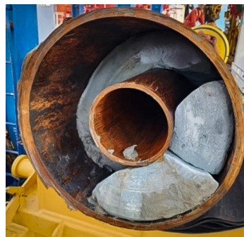
9 5 / 8 inch casing x 24 inch conductor cut
